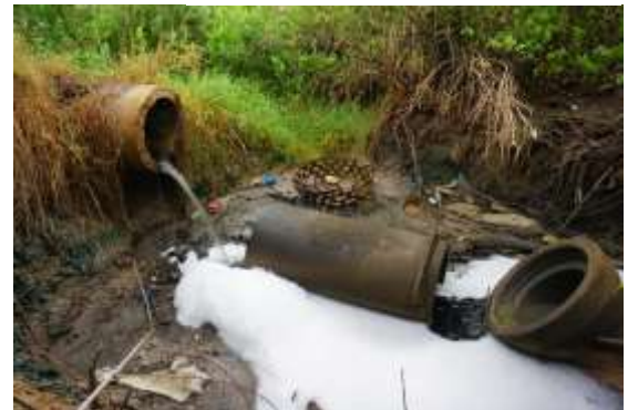
Photo 2. The discharge from Morogoro industrial Complex to the Ngerengere showing foaming as a result of untreated industrial wastewater. (Source: Water Witness)
