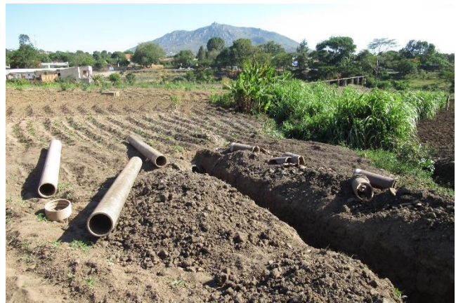
Sewage line repair
